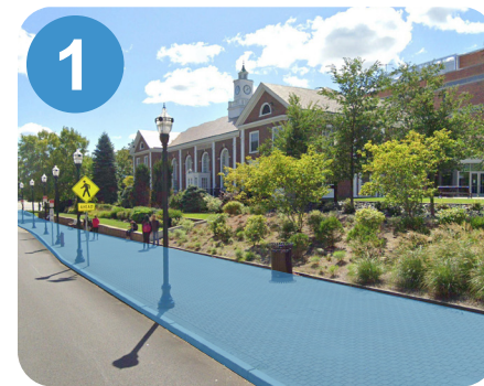
University Ave Pawtucketville's best sidewalks are along UMass Lowell's campus and are maintained by the university per their Master Agreement.
